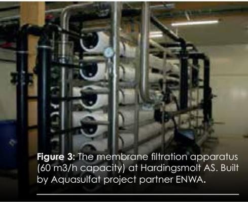
**Figure 3:** The membrane filtration apparatus (60 m<sup>3</sup>/h capacity) at Hardingsmolt AS. Built by Aquasulfat project partner ENWA.
